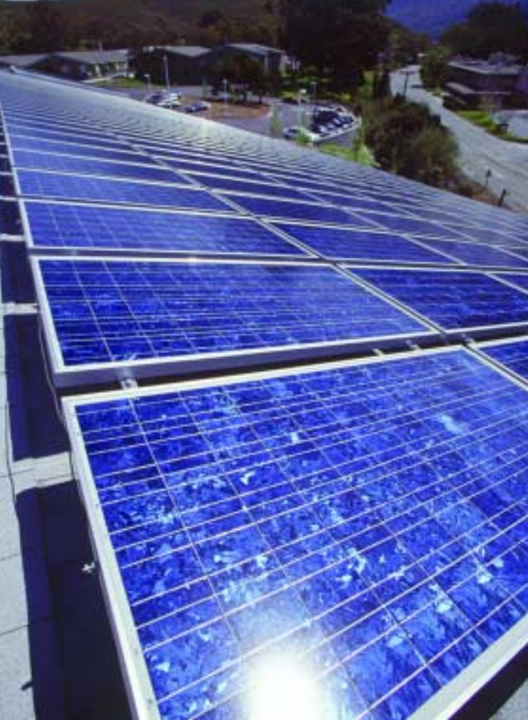
Roofs are angled to allow the PV panels to catch the sun, while overhangs shade the windows.
