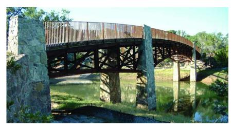
In designing the Spanish Oaks Golf Course Bridge at Hole #18, the landscape architect envisioned a structural steel pedestrian/golf cart bridge spanning over a man-made reflecting pond. The end result was a variable-depth arched-steel truss spanning to limestone-clad bents and abutments.
