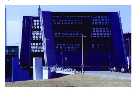
The Sixth Street Viaduct was a design-build project that replaced approximately 2,500' of bridge in downtown Milwaukee. The project includes two double-leaf bascules and two cable-stayed bridges whose design and construction were completed within just 24 months. Careful planning and coordination was required to meet the schedule for this complex bridge. The Sixth Street Viaduct is Wisconsin's first design-build project.
