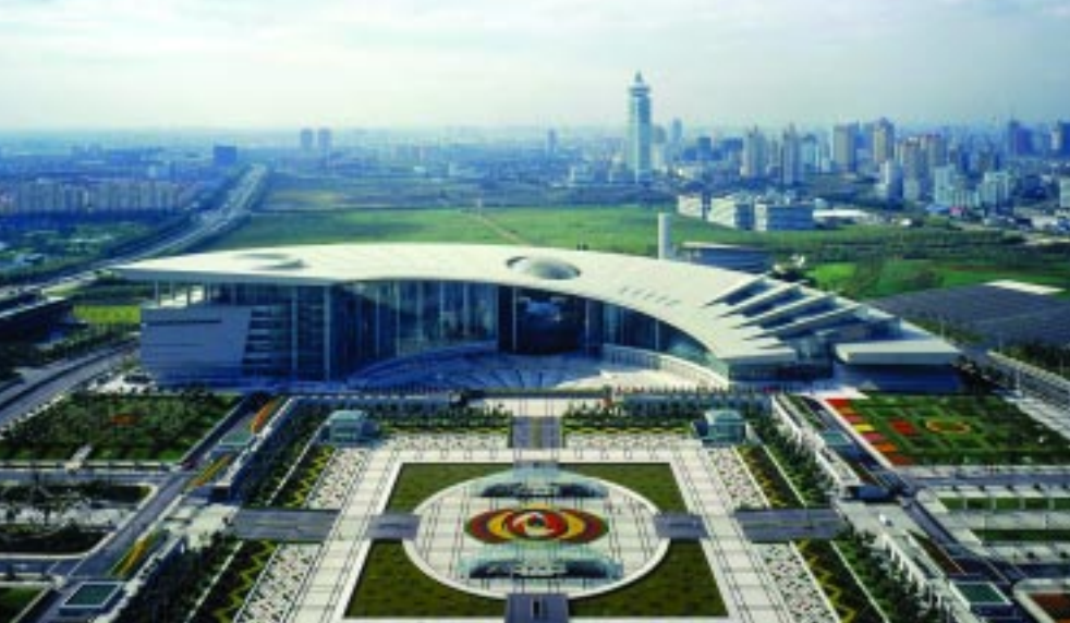
RTKL's asymmetrical design establishes a strong axis through the complex, which curves around the southern side of a civic plaza, and is located across from a government building, near Shanghai's Central Park.
