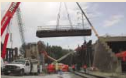
A part of the temporary bridge is lifted into place
