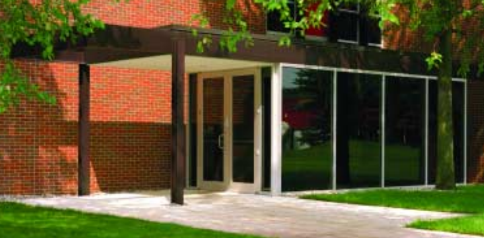
The new entry vestibule features an exposed welded frame of W6x15 columns and C15x33.9 beams in-filled with glass.
