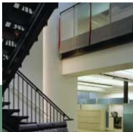
Old bulkheads at the balconies (left) were replaced with new, semi-transparent railings (right).
