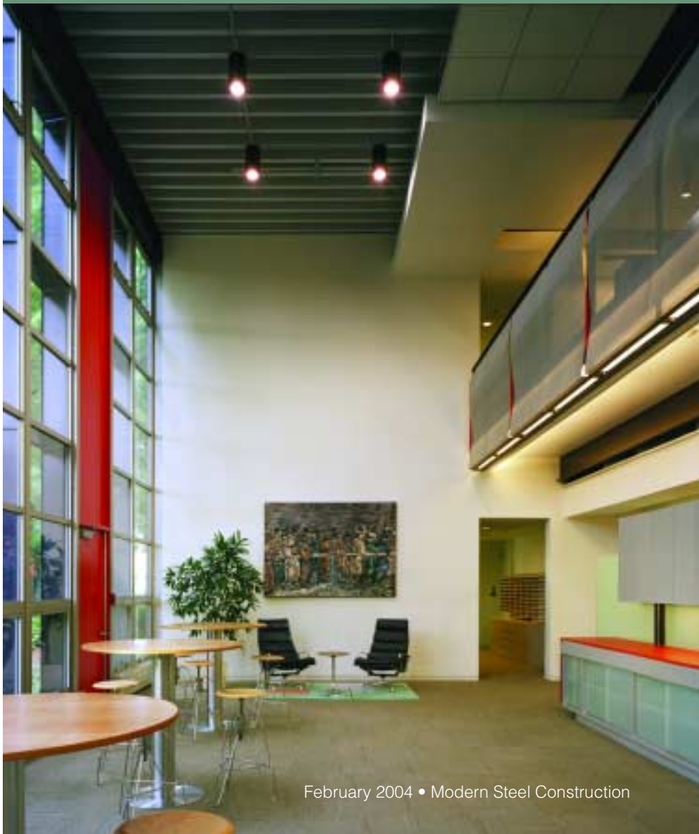
Below: New mezzanine balustrades of folded, perforated steel panels replaced the bulky fascias of the building's original interiors.
