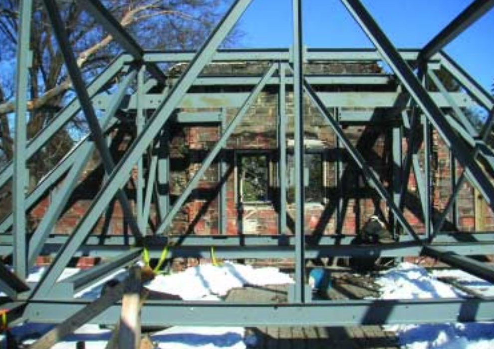
New roof trusses ( above ) made of C8s and L3x3s created the column-free interior spaces required for the gymnasium ( below ).
