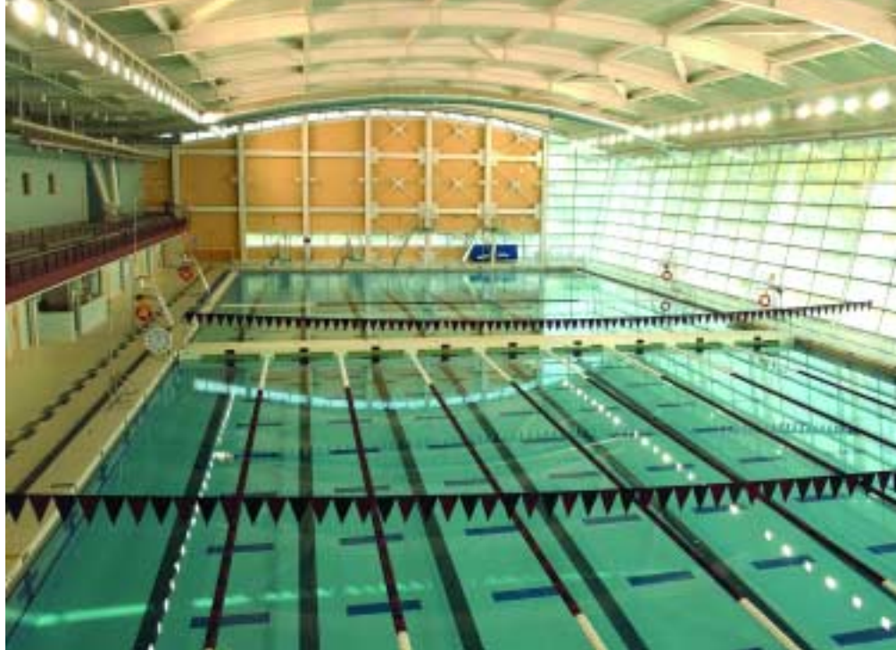
Both the natatorium (shown) and the gymnasium feature cable-supported roof structures.
