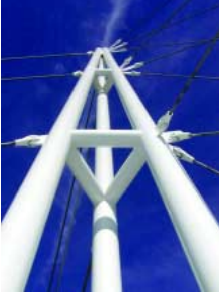
Above, left and right: The 10-story-tall masts are composed of three 18"-diameter steel hollow structural sections (HSS) arranged in a triangular, tapering form, and tied together with 12.75" HSS
