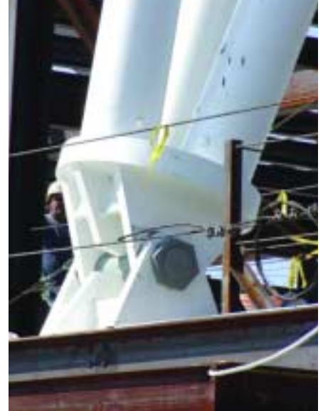
Pinned-base detail at masts.
