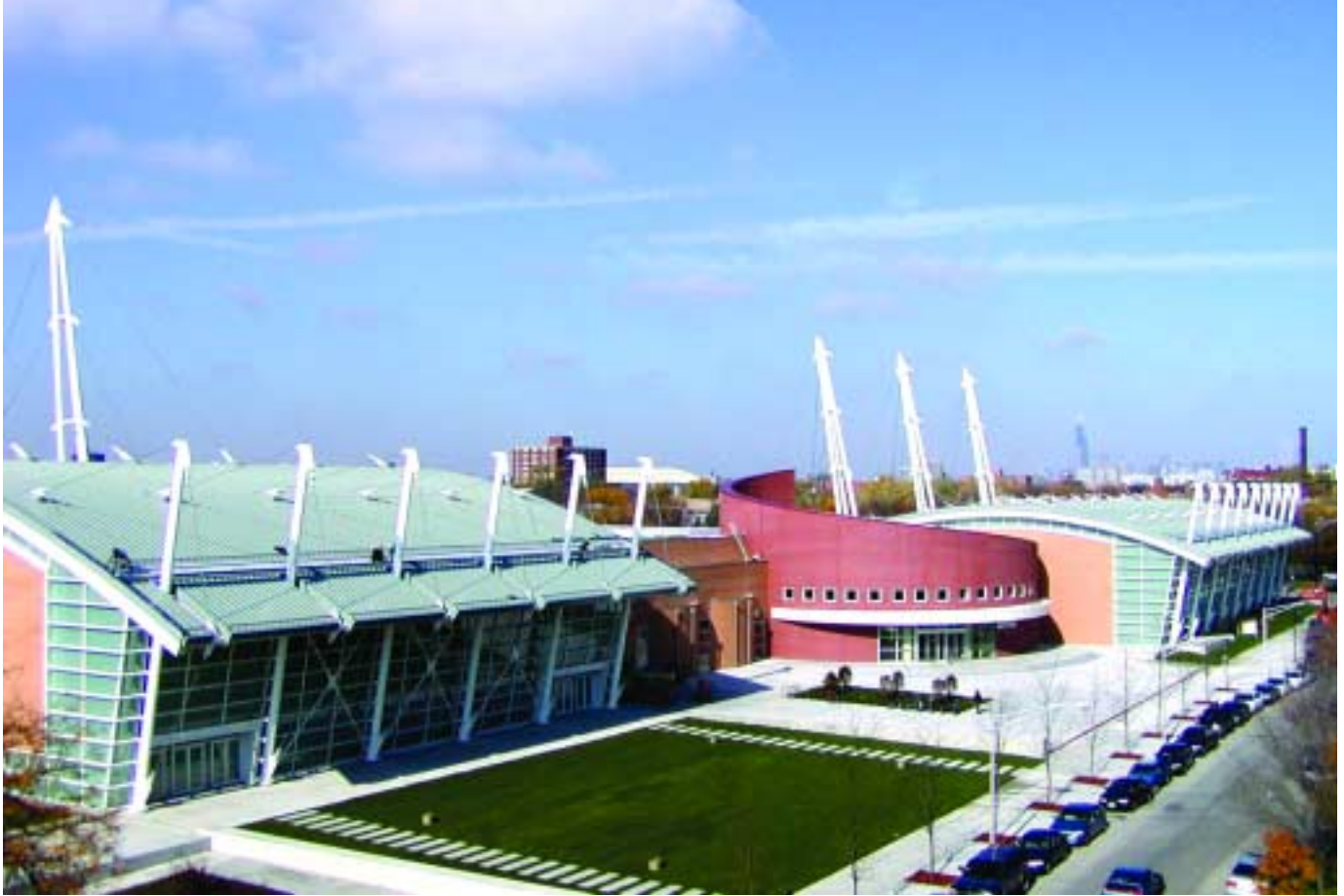
The Gerald Ratner Athletics Center at the University of Chicago consists of two asymmetrically supported cable-stayed buildings with multiple levels of splaying cables.
