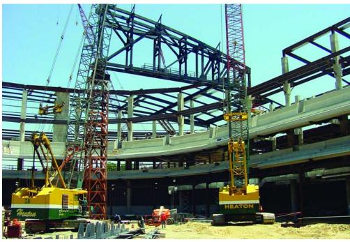
sense to have the truss bottom-chord elements serve double duty as rigging-grid beams. Likewise, W12 rigging-grid beams spanning east-west between the roof trusses also provide bottom-chord bracing for net-uplift conditions during a design wind storm.
