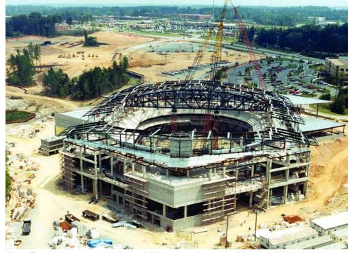
Above: The super-trusses exceeded normal shipping sizes. As a result, all connections are bolted so the truss could be assembled in the field. They vary in depth from 12' to 31'. Photo courtesy of Holder Construction
