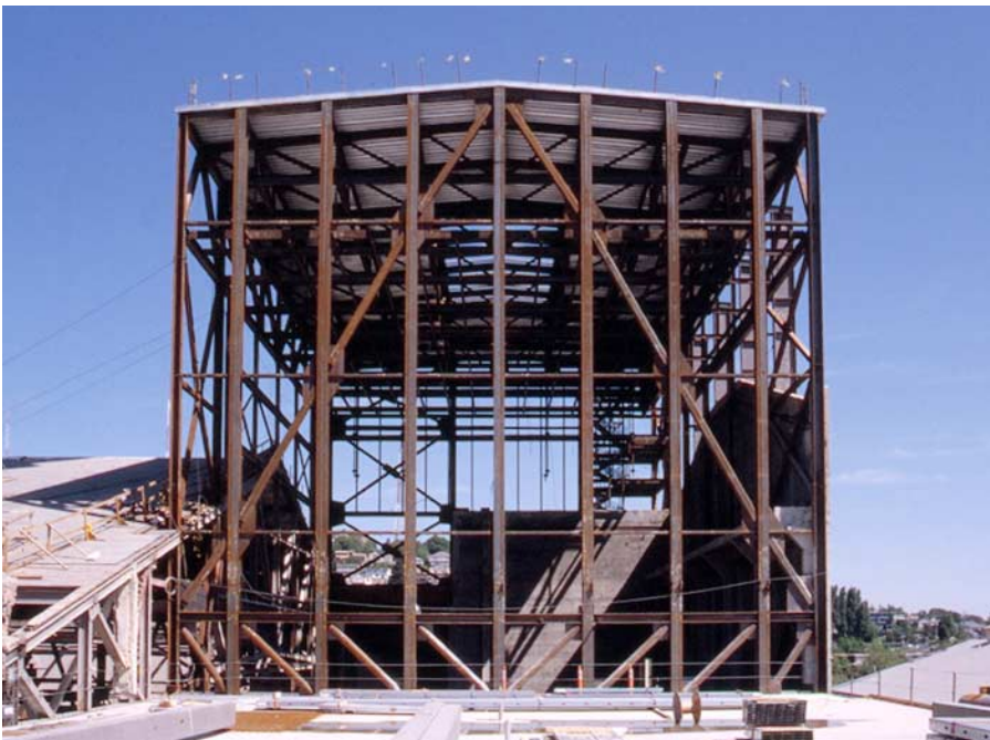
Above and below: New steel framing creates a larger fly loft to accommodate today's theatrical requirements. The peaked steel truss is part of the original 1927 roof structure. Drawing and photograph courtesy Michael Dickter and Magnusson Klemencic Associates.
