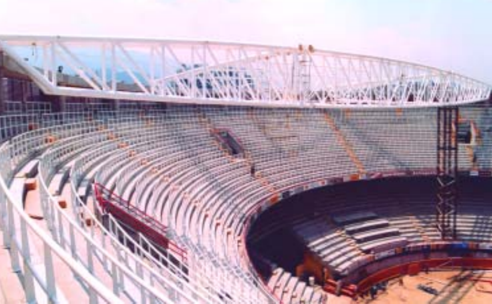
Each super-truss spans 233' and was shipped in six sections.
