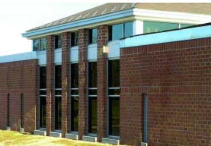
Below: Exterior view of the nearly completed structure.
