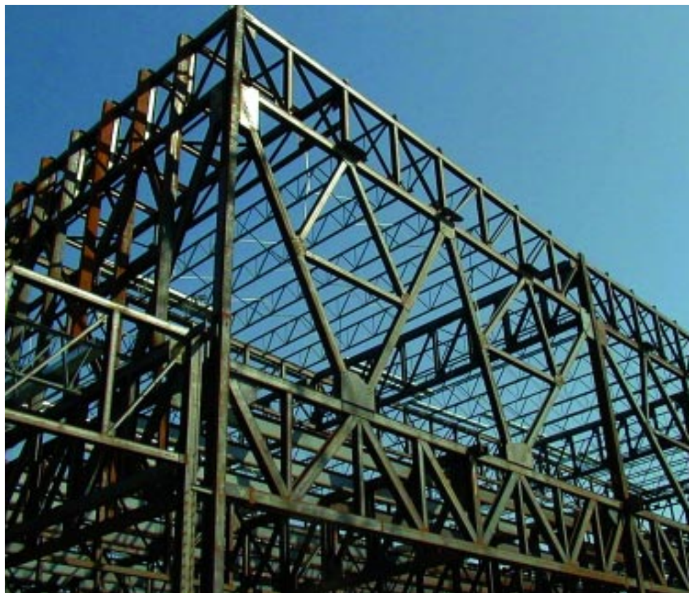
Below: Four 64'-deep truss systems, two floors in depth, were placed around the perimeter of the ballroom, shown here.
