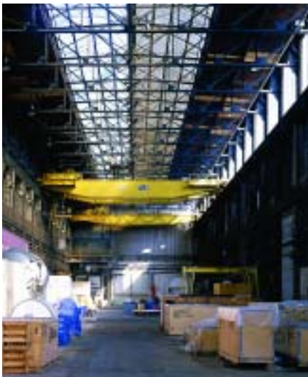
In their original configuration, the industrial buildings featured tall, open bays with bridge cranes.
