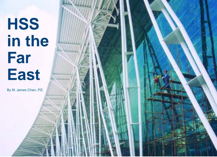
The main terminal features tilted and battered HSS columns of varying cross section, composed of three pipe shapes with plate stiffeners.
