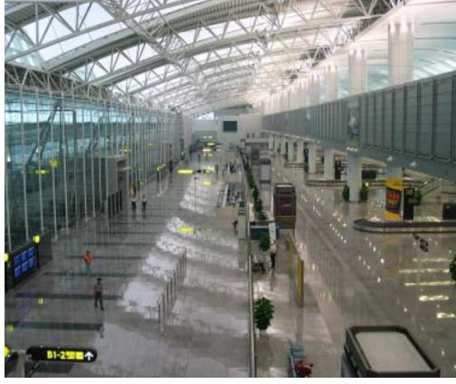
Triangulated trusses composed of round HSS create a dramatic interior space in the baggage claim area.
