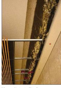
Figure 2. Example 2' 0" wide seismic joint
