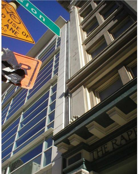
Seismic Joint Between Adjacent Buildings
