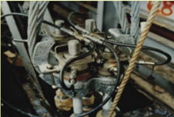
Bolting bridge support from the Williamsburg Bridge's main cable.
