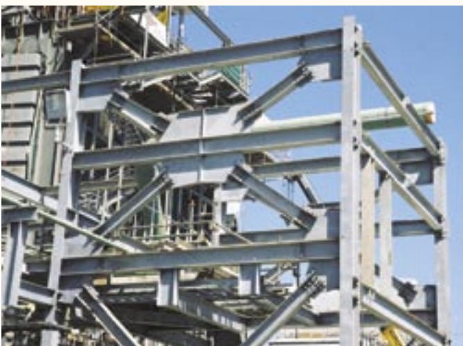
Steel-framed structure at a California power plant.
