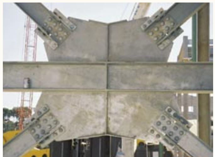
Typical braced-frame connection at a California power plant.
