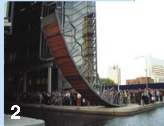
Figures 1, 2, and 3 show the sequence of the bridge unrolling after being opened to allow passage through the canal.
