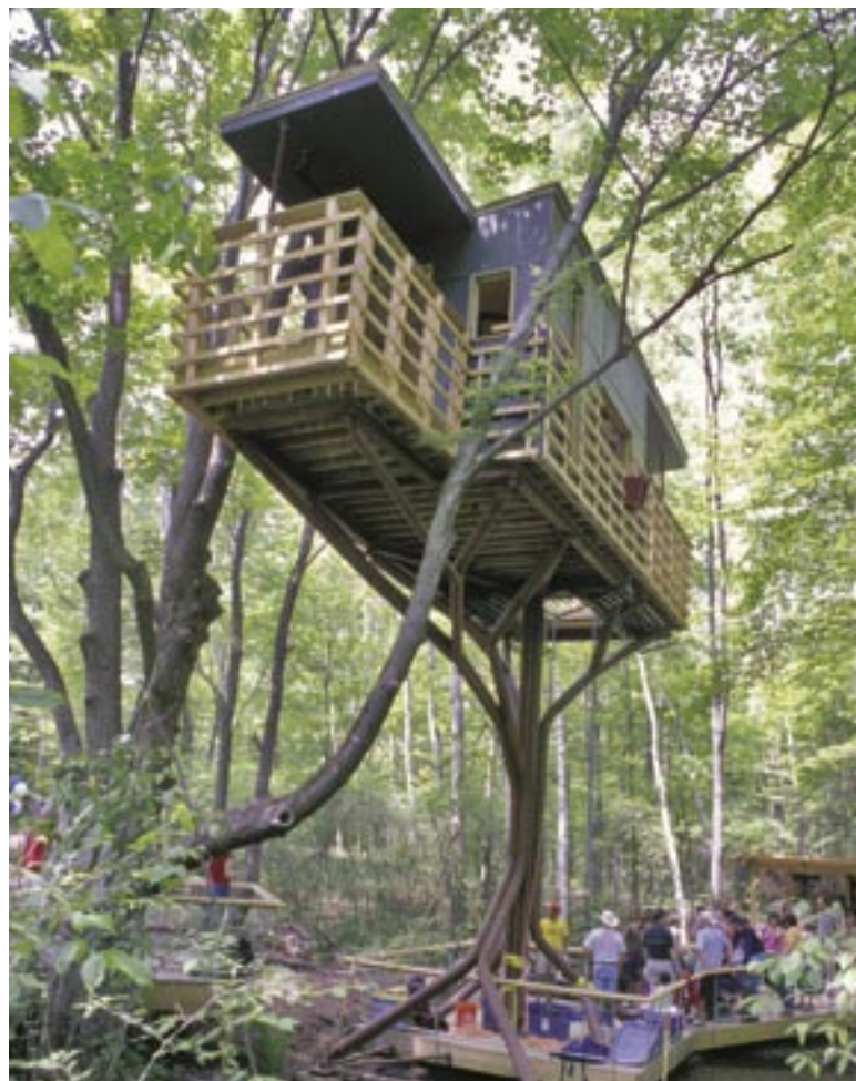
Because of poor soil conditions at the site, the tree branches downward (as well as upward) to counteract the eccentric loading of the tree house. Photo by Peter von Buelow.
