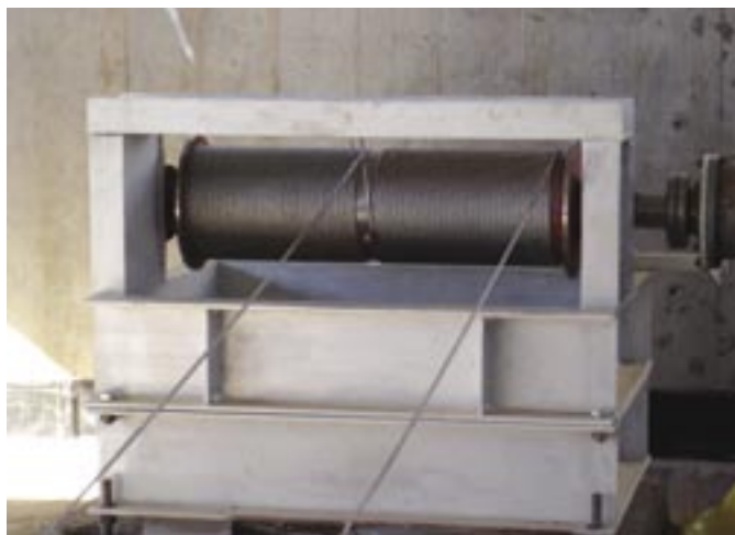
An electric-driven winch spools the cables that pull the roof forward and backward.
