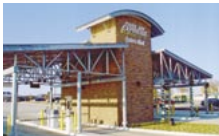
Park Air Express (Irving, Texas), transportation category winner, was galvanized by AGA member and AISC associate member Aztec Galvanizing Services—Crowley of Fort Worth, Texas.
