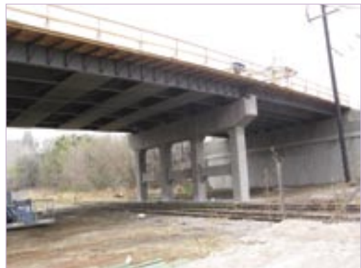
The new viaduct (above) over the railroad tracks features full-width blast plates salvaged from the original bridge (below).
