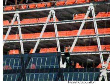
The engineer had actually designed the plates with four pieces of 5" plates welded together to build these bird's mouth nodes, but we ended up coming up with a design to use two 10"-thick plates. There were 84 of the internal 10" nodes and 16 of the bird's mouth nodes.
