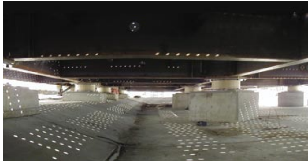
Above and Below: Seventy-six high-damped rubber elastomeric bearings made by Bridgestone Rubber of Japan function as part of a base isolation design that keeps building accelerations below 0.5 g even in worst-case analyses.
