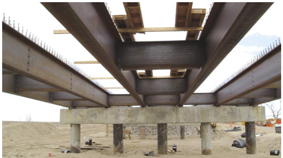
Roller beam girders and diaphragms form the steel superstructure for the bridge.
