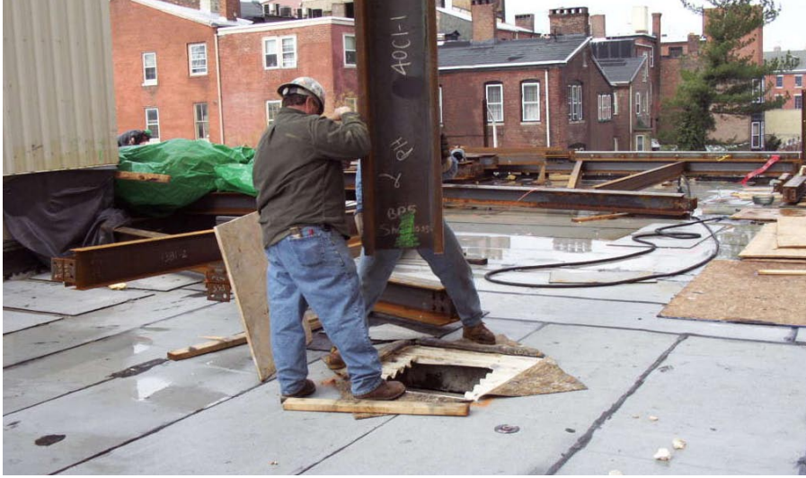
New columns were threaded through small openings in the existing structure.
