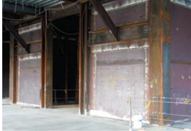
Above: In locations where the code-prescribed aspect ratio of the steel plate panel was not naturally achieved, KPFF added intermediate horizontal boundary elements (HBEs) with wide-flange steel kickers between floor levels.
