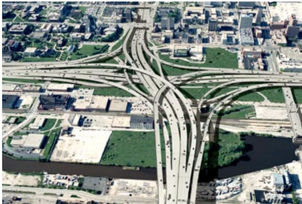
A rendering of Milwaukee's Marquette Interchange in its reconstructed form. The interchange will connect I-43, I-94, and I-794. Courtesy WisDOT.
