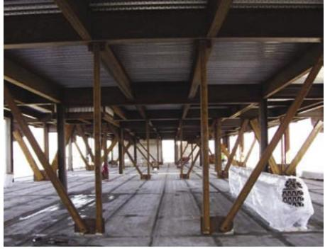
View of the 16th floor. The staggered trusses at this level are fairly light, because there are few supported levels above. Composite beam and girder framing was used for the 17th floor slab and upper mechanical penthouse levels.
