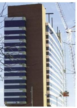
Forty-six story-high, 7-panel, Pratt-style staggered steel trusses were used in the tower to frame the fourth through the 16th floors. Due to the unsymmetrical nature of the offset curved long faces of the tower, each staggered truss had a slightly different length and geometry.
