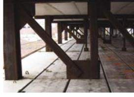
Staggered trusses were framed into the walls between hotel rooms. Floors are framed with 4-ft-wide, 10-in.thick precast prestressed concrete planks. The planks span 30 ft between the bottom chord of one staggered truss and the top chord of the next.
