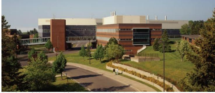
The skywalk structure (far left, above) consisted of trusses spanning approximately 76 ft with an 8-ft cantilever near the existing building.
