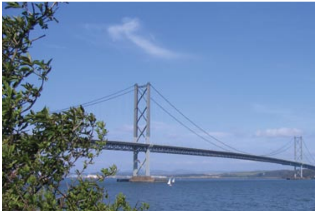
The cables on Scotland's 3,300-ft-long Forth Road Bridge were recently inspected for damage.
