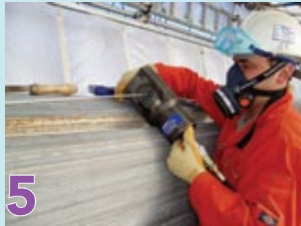
New wires are installed as necessary.
