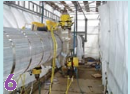
The cable is recompactified...
