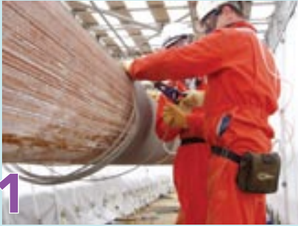
The existing wrapping is removed from the cable.
