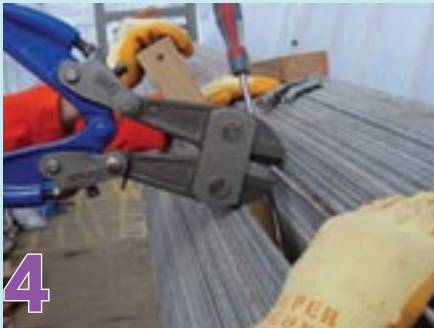
A sample wire is cut and tested.
