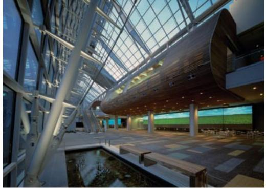
Vertical "fishbone" trusses (at left in photo)—consisting of round HSS, cruciform cross-section arms, and tension cables—support the glass enclosure of the pre-function space.
