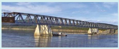
ery and erection schedule. This includes the deck steel, railings, and structural steel. The bridge is comprised of three spans in excess of 400 ft each, as well as about one-half mile of approach causeways.
