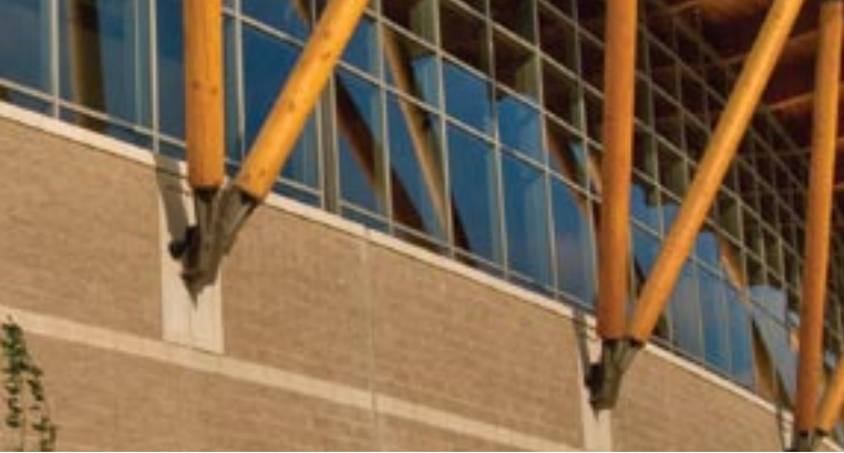
The V-braces punctuate the exterior of the 900-ft-long serpentine concourse.
