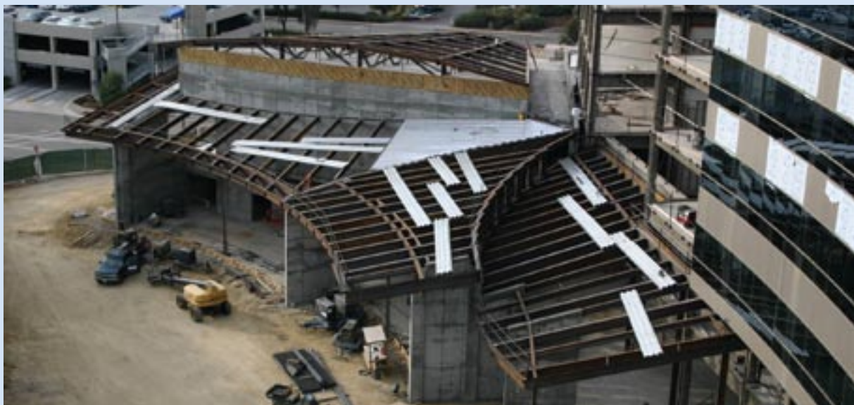
Overall construction view of lobby and lecture hall steel roof framing.
