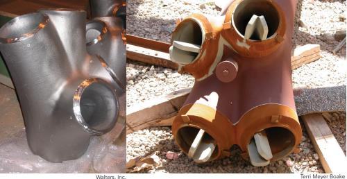
the tree carry the loads from the grid-like wide-flange framing system that supports the atrium roof, down through its tubular trunk to the concrete foundation below. This type of geometry, in its tree-like stretch, creates large eccentric forces that put significant moment stresses into the nodes connecting the branches.
