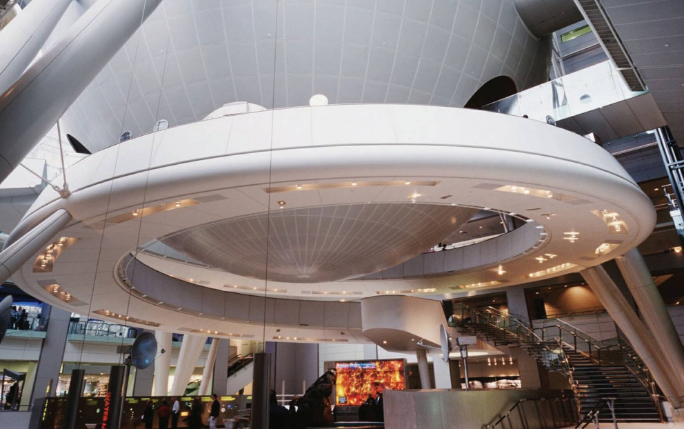
Projects such as New York's Hayden Planetarium, with its unique design and large amount of exposed steel, make attractive fireproofing a necessity. Photo: Polshek Partnership Architects
