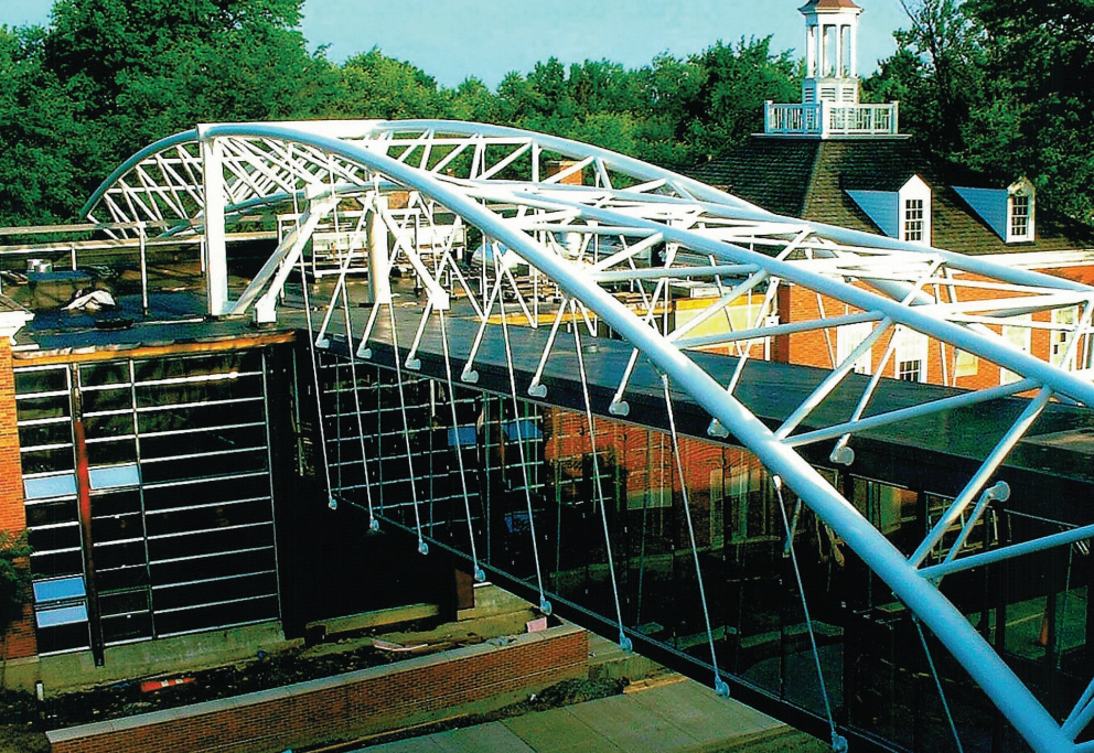
The glass walkway of the Cleveland Heights – University Heights Public Library features HSS prominently in its exterior trusses.
