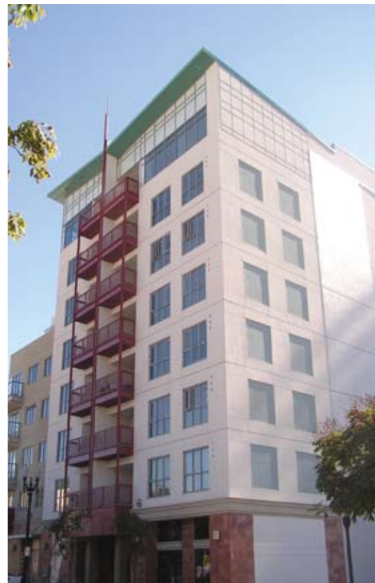
Painted galvanized steel was used for Nexus' balconies.
