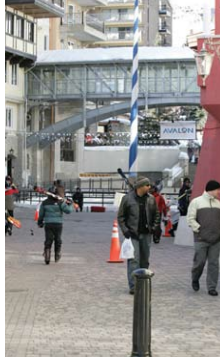
The completed pedestrian bridge, ready for skiers.
