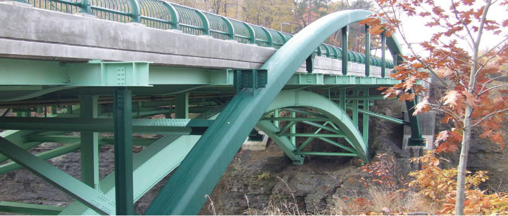
Existing and new steel framing elements were painted light green and dark green, respectively, to provide differentiation between these elements.
