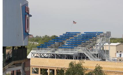
The bleacher system's beams and columns sit on the building's existing load-bearing masonry walls and a new concrete roof (left). From across the street from Wrigley Field, 200 fans can get a clear view of the action (right).
