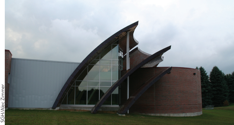
View of the south façade of the Michael Klahr Center, showing all four petals.
