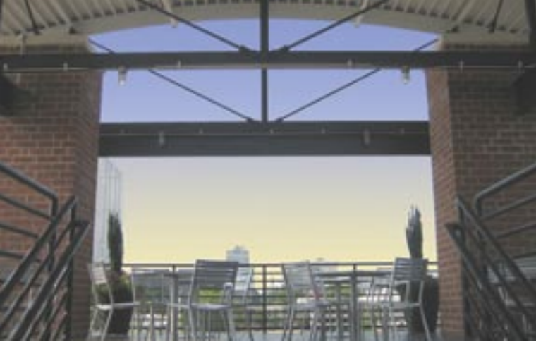
A new two-story entry to the complex (shown from the interior, left, and the exterior, right) showcases trusses and a curved roof, hinting at the bow-truss roof inside the converted buildings.
