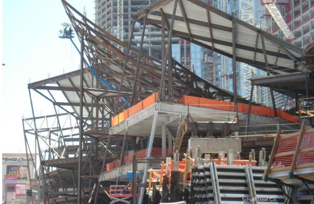
The weights of the various trusses range from 5 to 90 tons.
