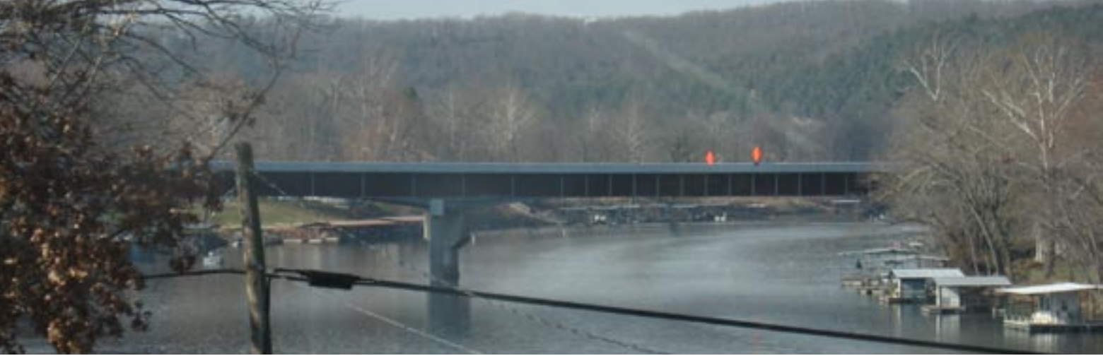
The two main spans are 230 ft long, and the bents were skewed at 20° to match the river's flow.
