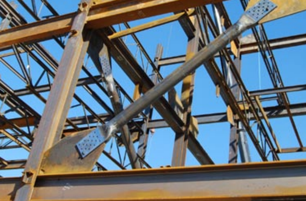
An SCBF with round HSS bracing equipped with High-Strength Connectors.
