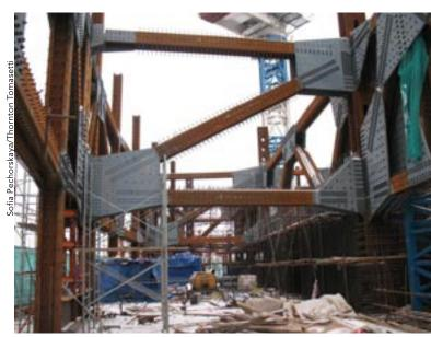
The west section of the 33rd-floor outrigger trusses, linking the belt truss on the left to the central core on the right. JULY 2009 **MODERN STEEL CONSTRUCTION**
