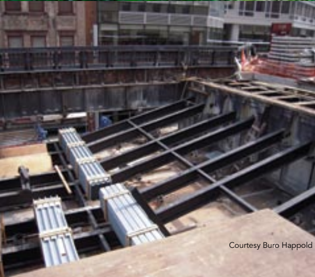
A view of the 10th Avenue Square portion of the project, with the pre-existing slab removed. Bleachers overlooking the street were being installed at this point.
