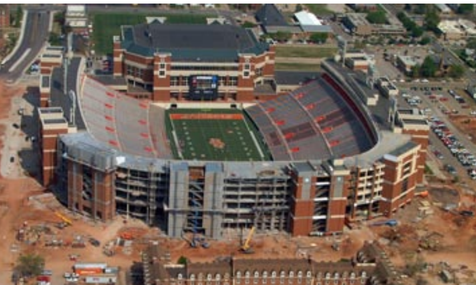
The Boone Pickens Stadium expansion used 10,000 tons of structural steel. MODERN STEEL CONSTRUCTION AUGUST 2009
